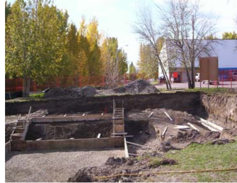
Putting in the forms
