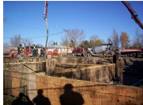
Pouring concrete into the forms
