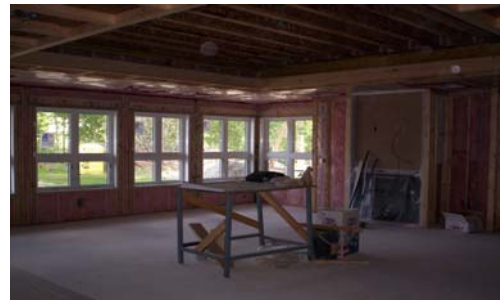
Work station set up inside
