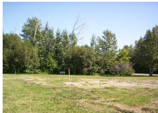
Readying site to begin building
