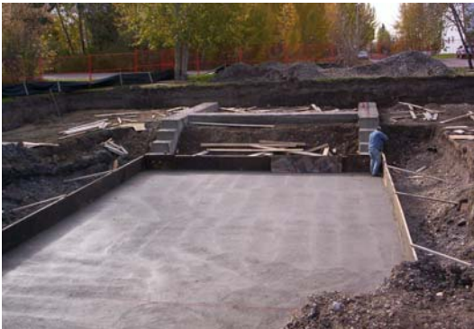
Preparing to wrap the concrete pad
