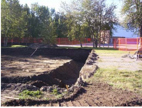
Digging for the foundation
